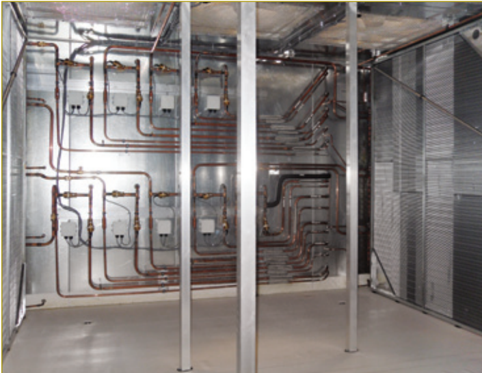
Interior of a 180 ton ACCU that has easy access to all refrigeration piping and components.
