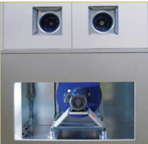
Example of a single fan airflow supply with smaller dual return airflow fans to accommodate height restrictions.
