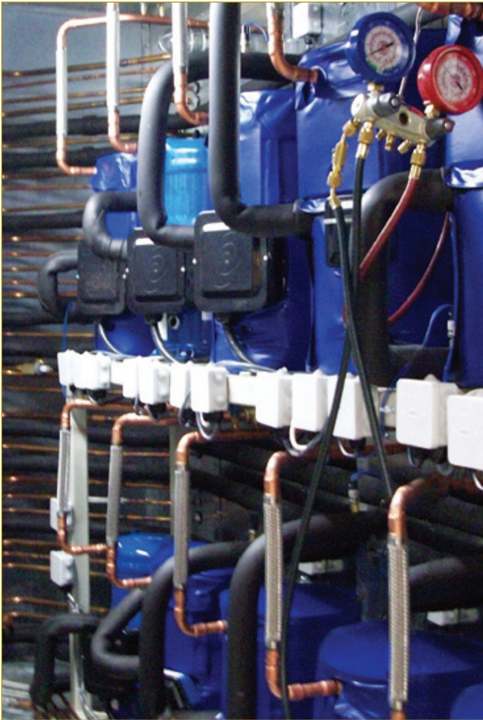
Example of an integrated 160 ton ACCU with a 7 ft. wide vestibule for compressor, control panel, receivers, sight glass and VFDs.
